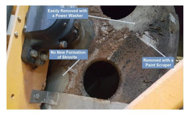
**Image 3** – HydroFLOW has Prevented New Struvite and Caused Easy Removal of Existing Struvite
